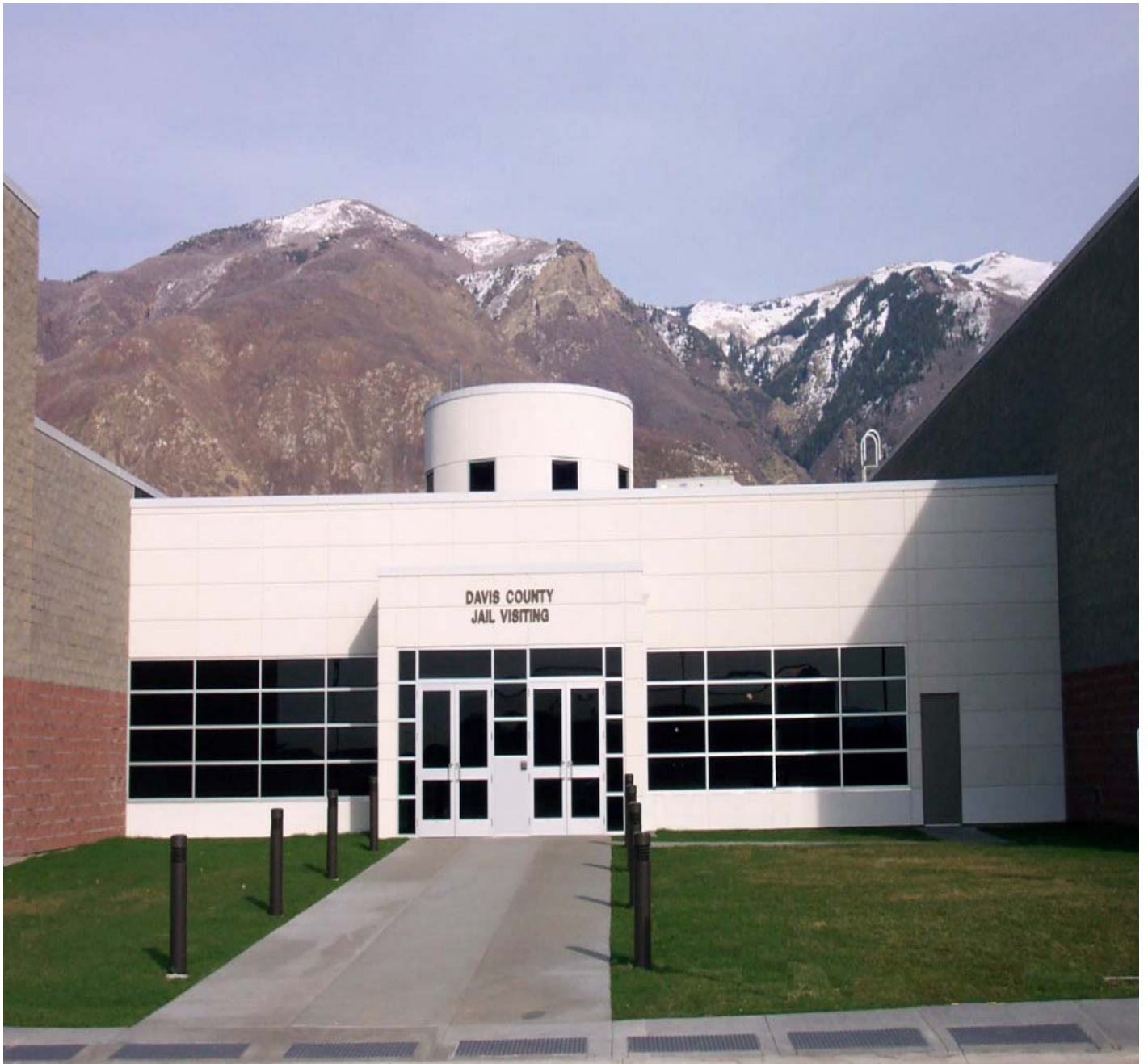
Davis County Jail Expansion, Farmington, Utah
